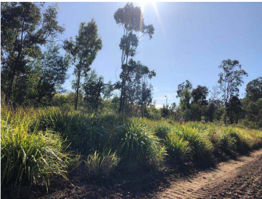
Photo set 9: Improvement works within Lots 7002 and 7003, now off-maintenance.
