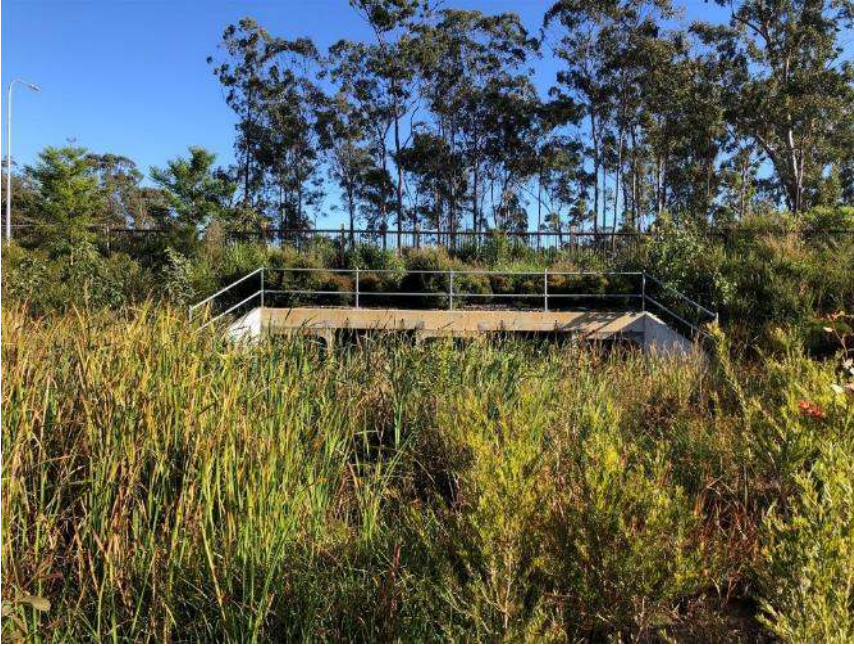
Photo 5: Native flora regeneration at the entry of the culvert underpass.
