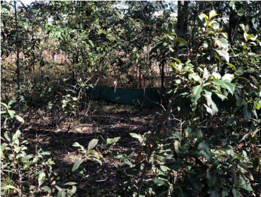
Photo set 3: Fauna friendly and erosion and sediment control fencing.
