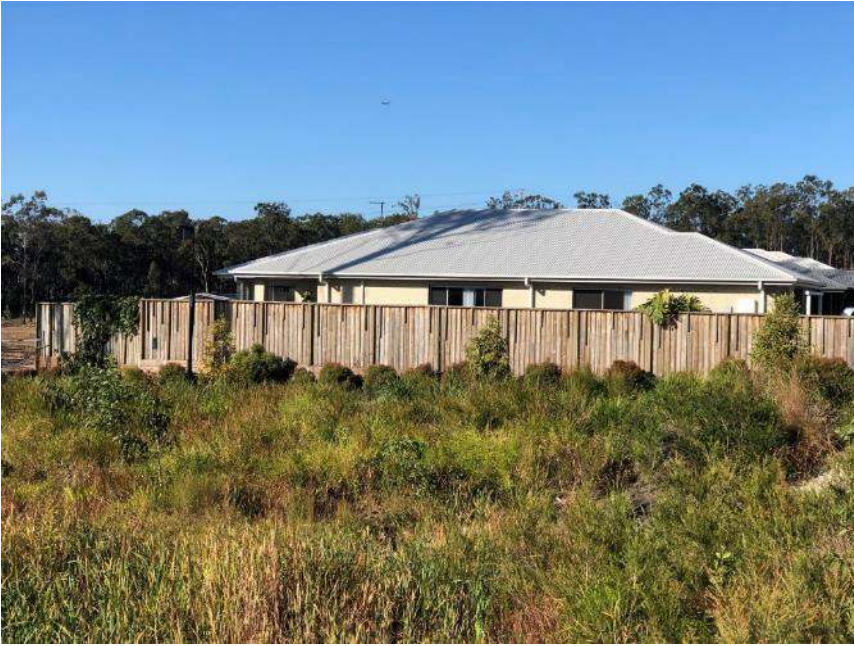
Photo 7: New build residence with fauna exclusion fencing, adjacent to the drainage and stormwater conveyance corridor.
