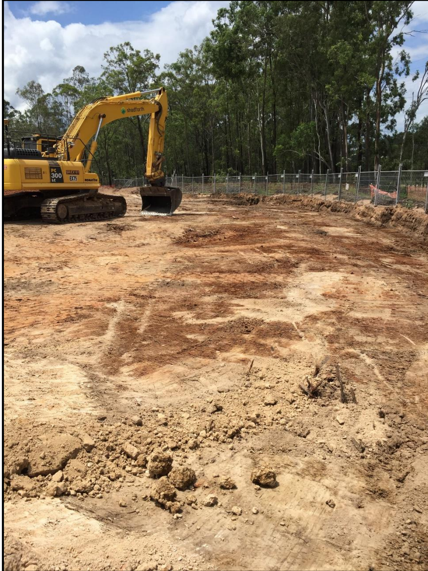
Picture 2: View of Stripping Operations
