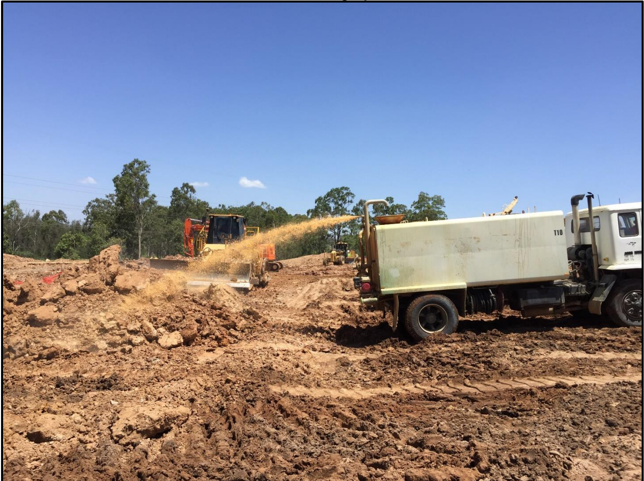
Picture 3: View of Filling Operations
