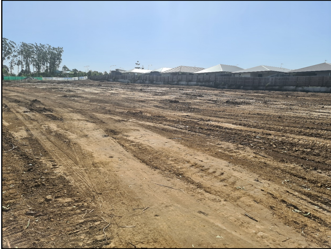
Picture 2: View of Stripping Operations
