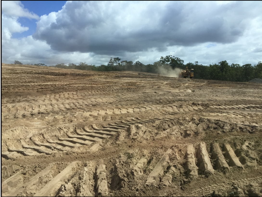
Picture 2: View of Stripping Operations
