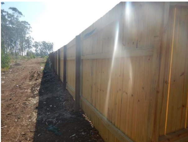
Image 6: Koala exclusion fencing interface between residential development and the Goodna Creek open space area
