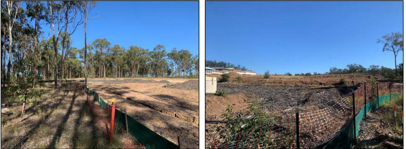
Photo set 1: Fauna friendly and erosion and sediment control fencing.
