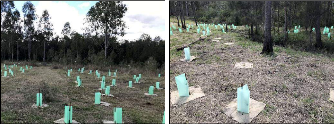
Photo set 2: Improvement works within future Lot 7004 (June 2021).
