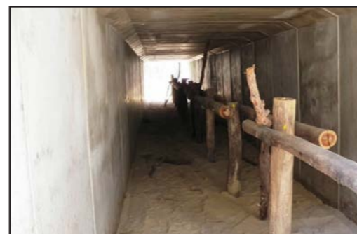
FAUNA CULVERT WITH RAISED LOG ACCESS
