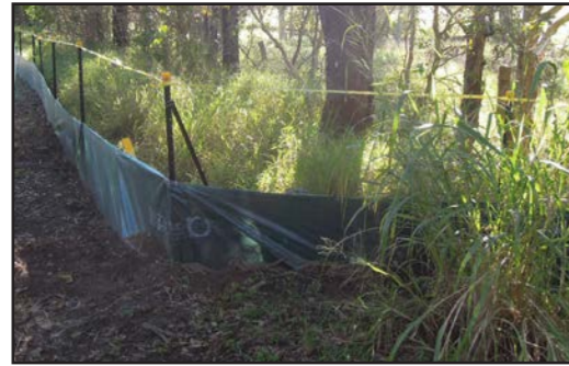
TREE PROTECTION & EROSION FENCE
