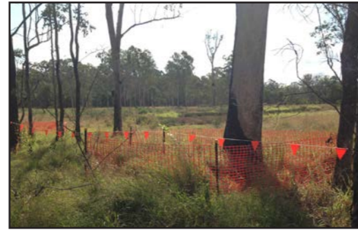
SIGNIFICANT TREE PROTECTION FENCING
