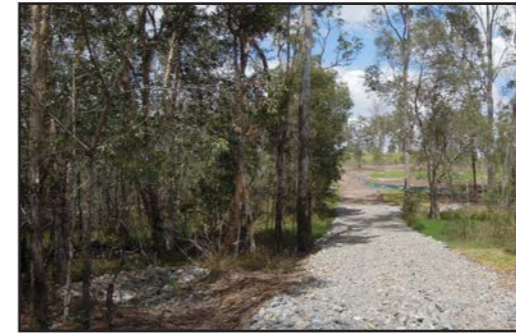
CONTROLLED CLEARING ACCESS TRACK
