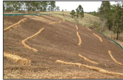
EROSION CONTROL TO CLEARED BATTER
