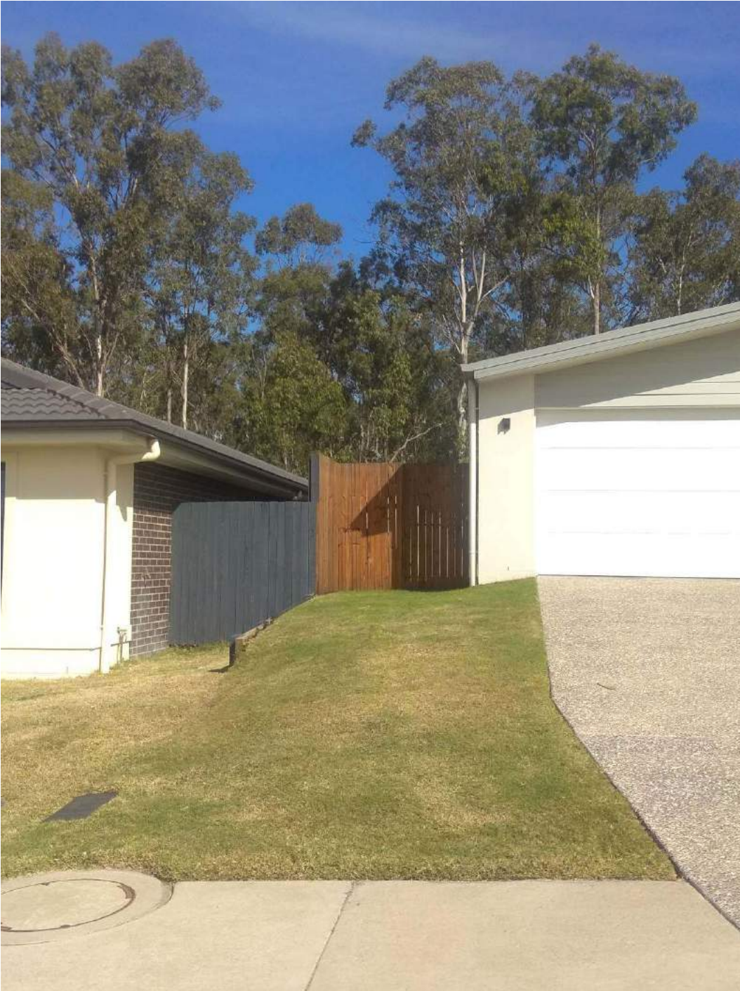
Image 3: Fencing prevent koala access to backyards
