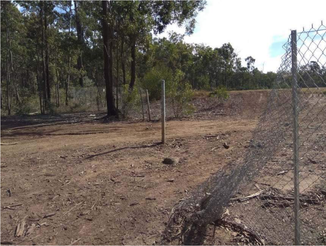
Image 8: Illegal access to the detention basin
