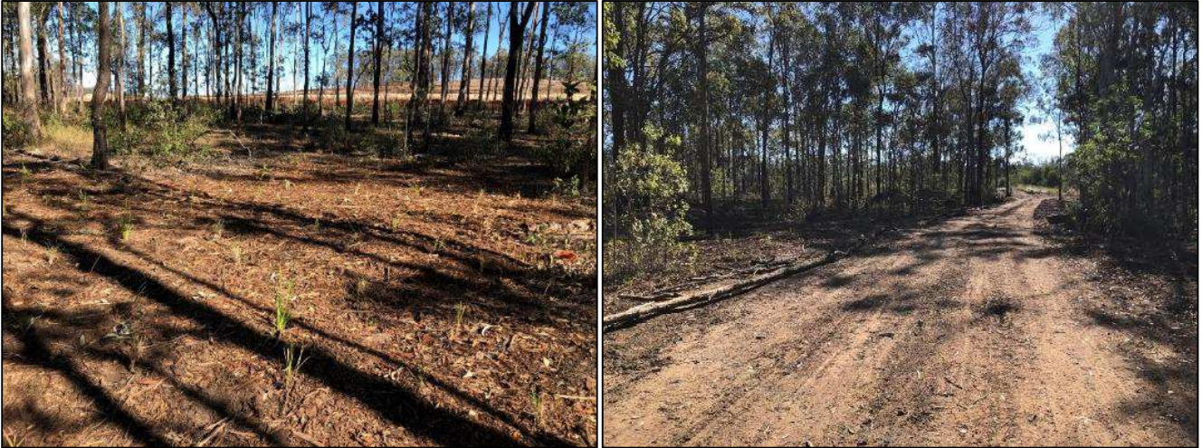
Photo set 1: Improvement works from Lot 7002 and 7003 following practical completion.
