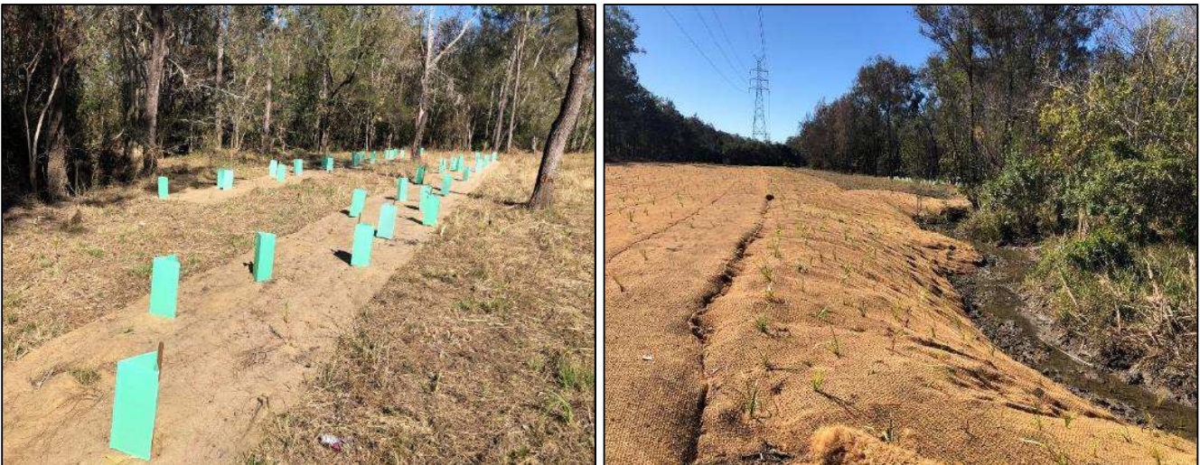
Photo set 2: Improvement works from Lot 7002 and 7003 following practical completion.
