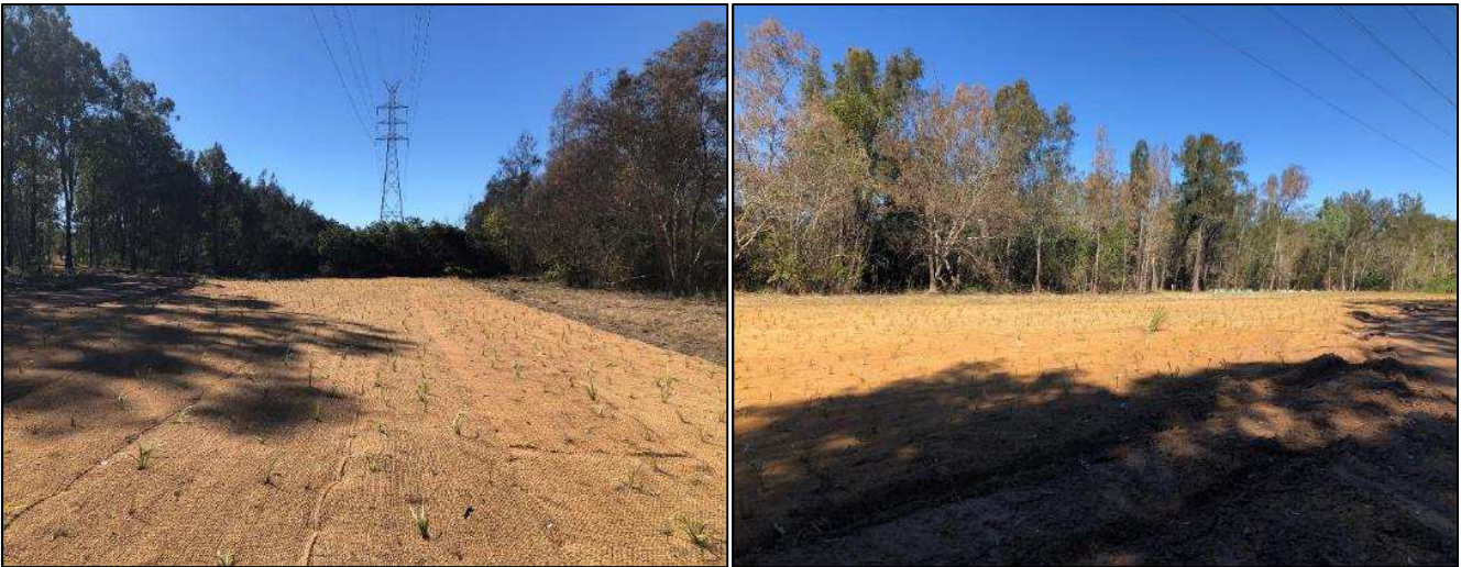
Photo set 3: Improvement works from Lot 7002 and 7003 following practical completion.
