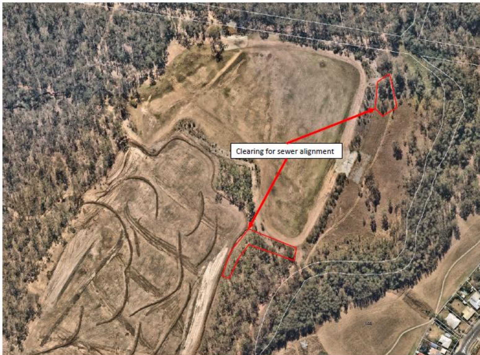
Figure 2- Extent of clearing- Sewer Alignment
