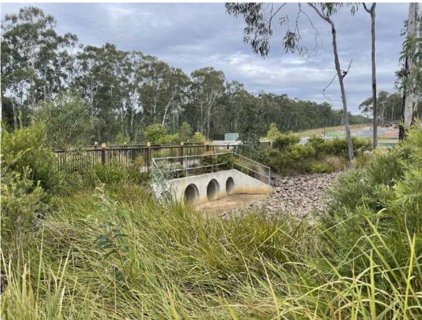
Photo 2: Native flora regeneration at the entry of the culvert underpass.
