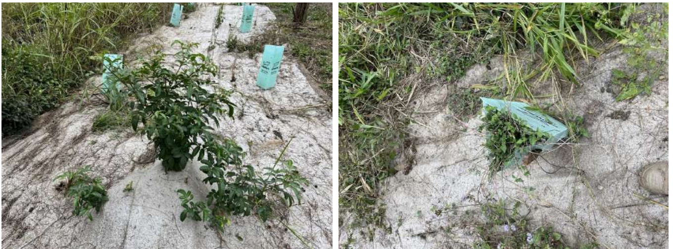
Photo set 7: Weeds dominating geofabric ground cover and inside tree protection sleeves in lot 7003.
