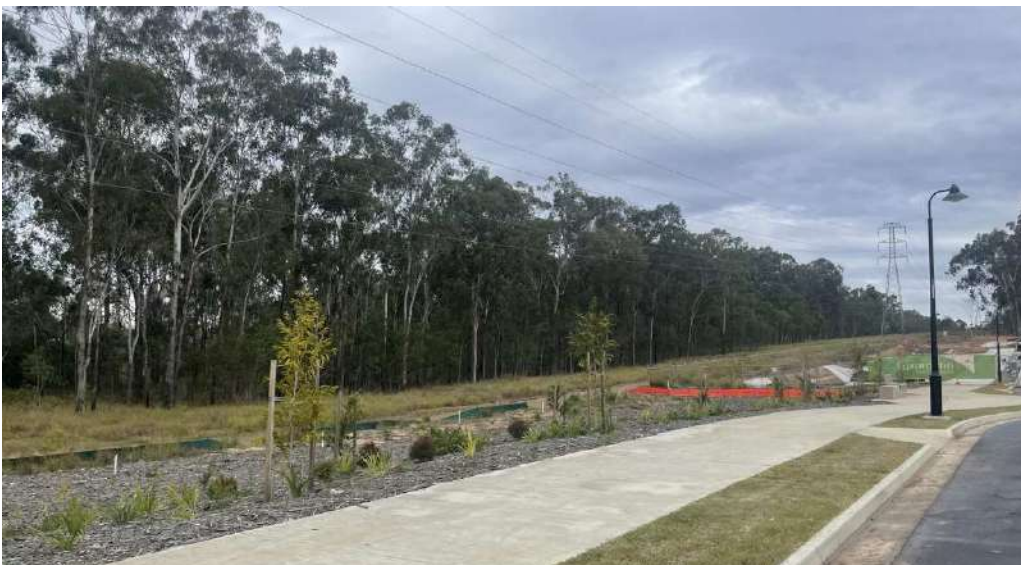
Photo1: Erosion and sediment control fencing on clearing extents post-earthworks.
