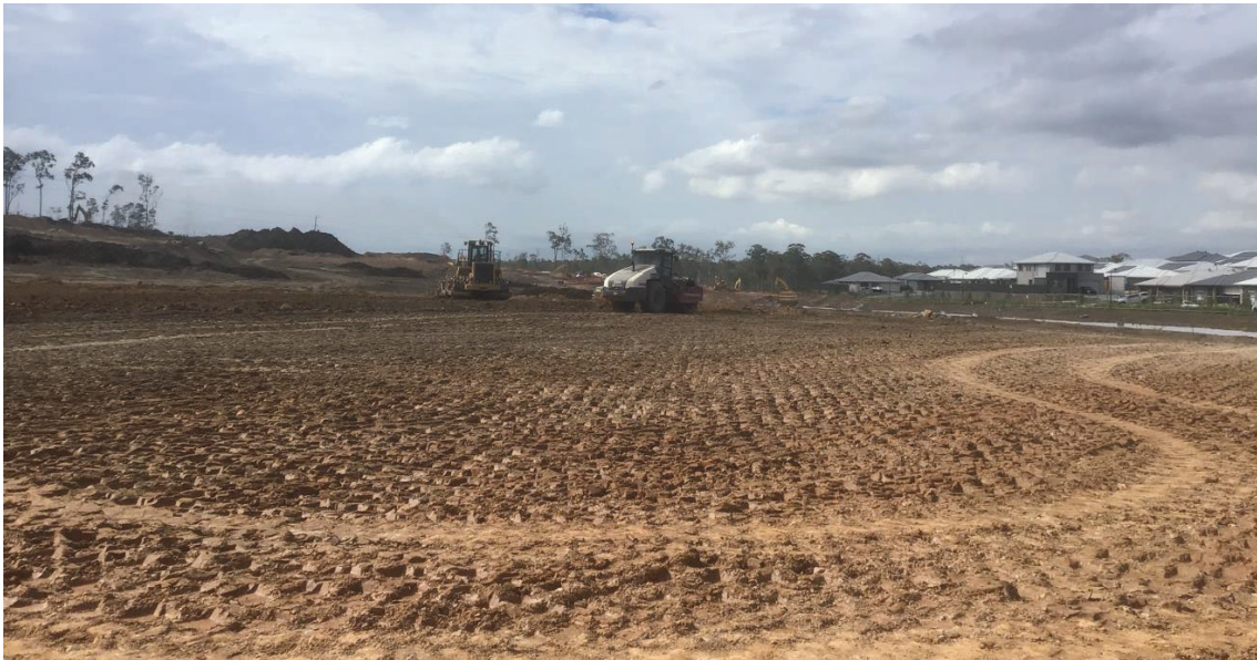
Site Image 2 – Filling Operations in Progress
