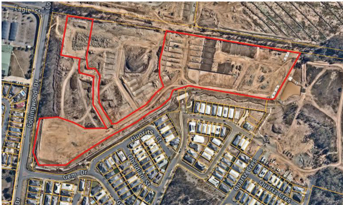
Figure 1: Approximate Extent of Level 1 Works (Image from Nearmap ©)
