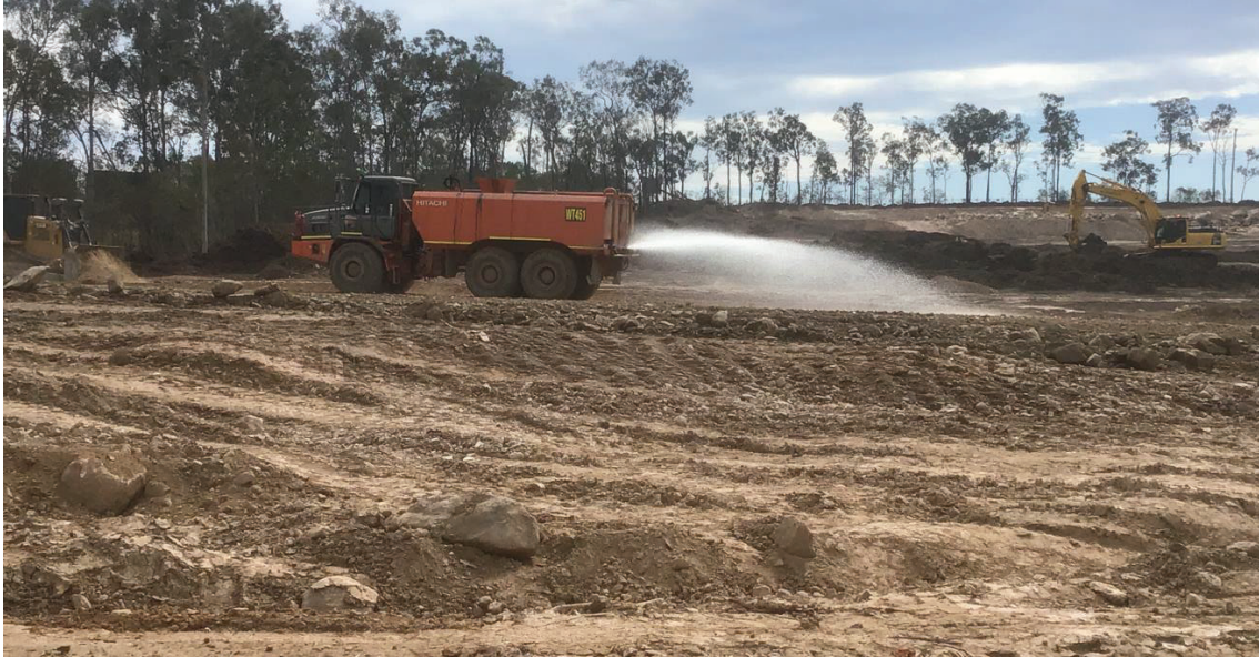
Site Image 1 – Filling Operations in Progress
