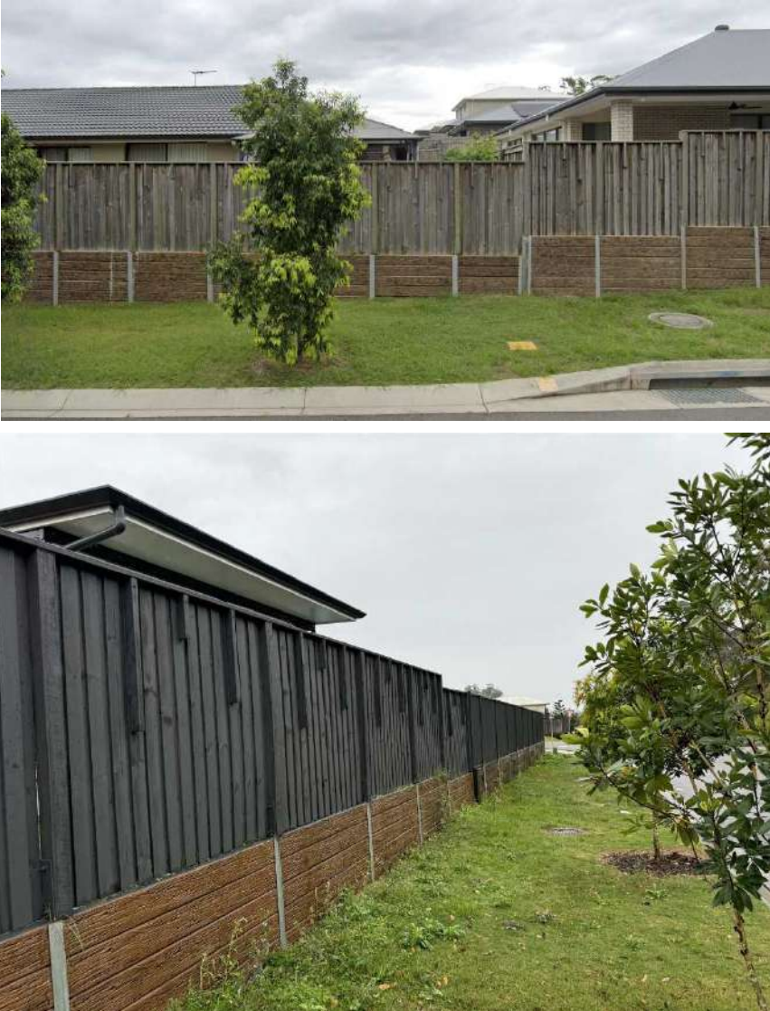
Photo Set 4: New build residence with fauna exclusion fencing adjacent to rehabilitated areas.
