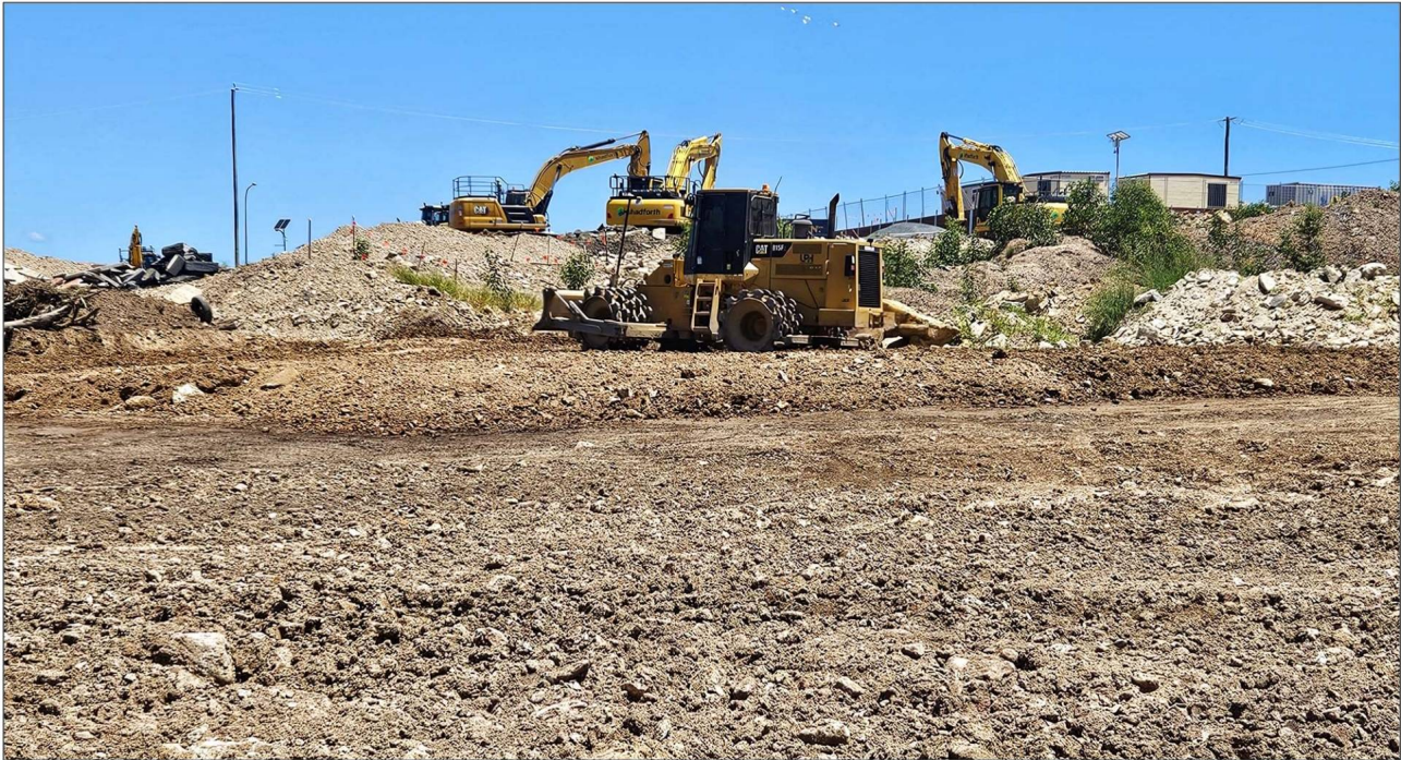
Figure 4: Compaction and proof rolling operations in progress – (28/01/2025)
