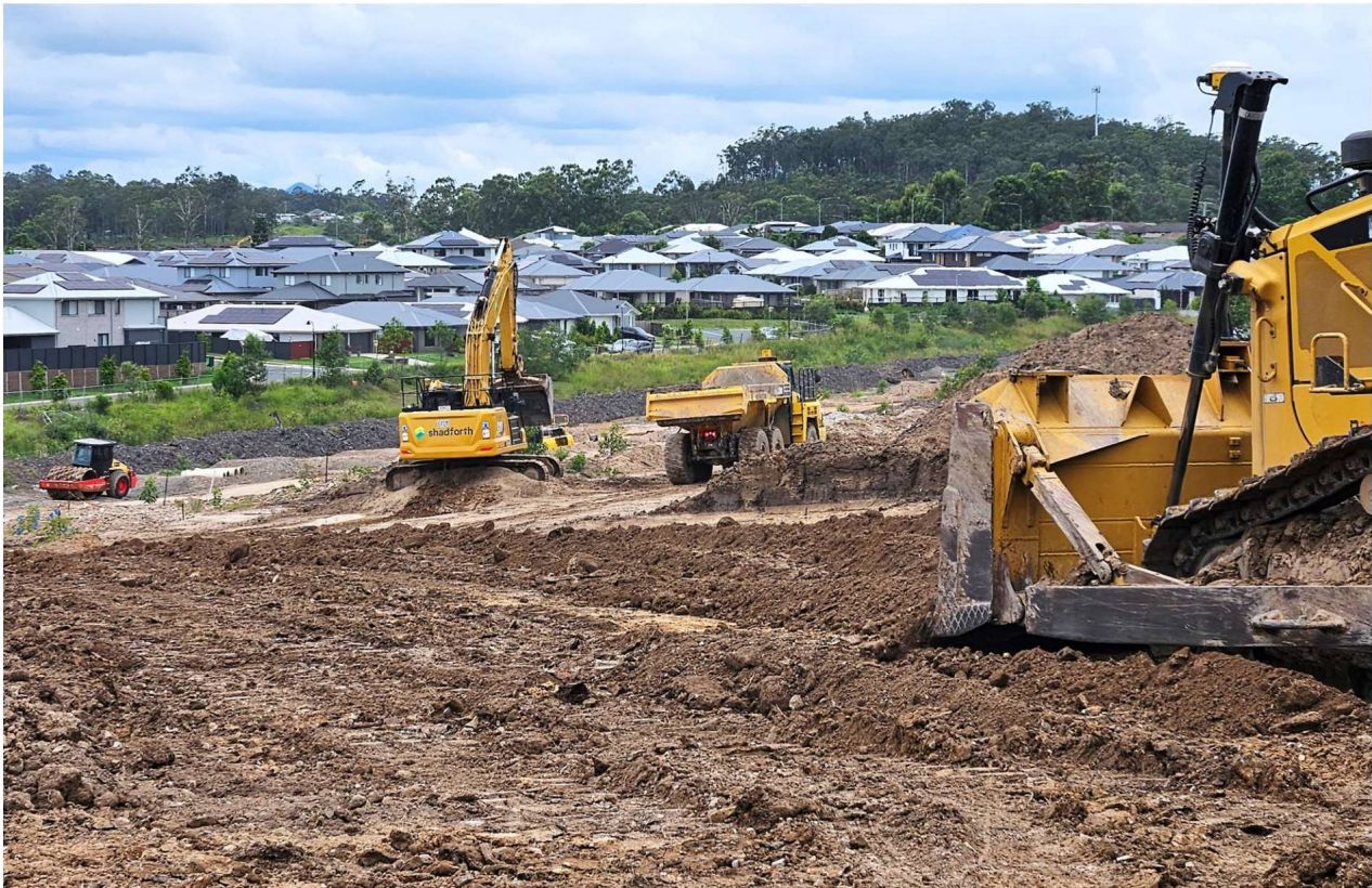
Figure 3: Filling and compaction operations in progress – (15/01/2025)
