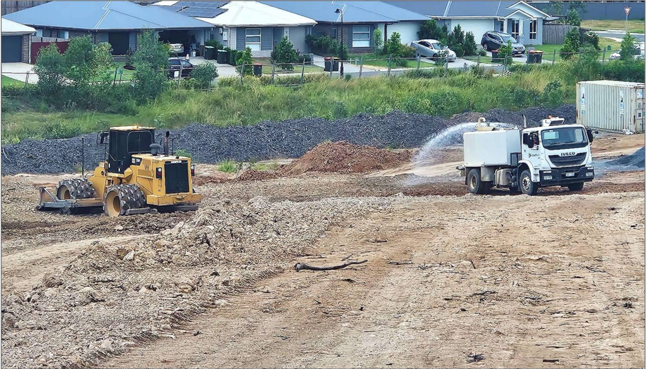
Figure 5: Compaction and moisture conditioning operations in progress – (05/02/2025)
